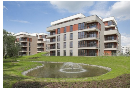
Ostoja-Wilanów (stage 2). Date of delivery: 2009 No. of units: 221 apartments (19,944 sq. m). 4 commercial units (600 sq. m).
